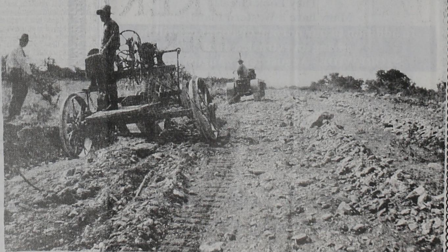
Men at work building roads south of Roaring Springs, 1933-34.
