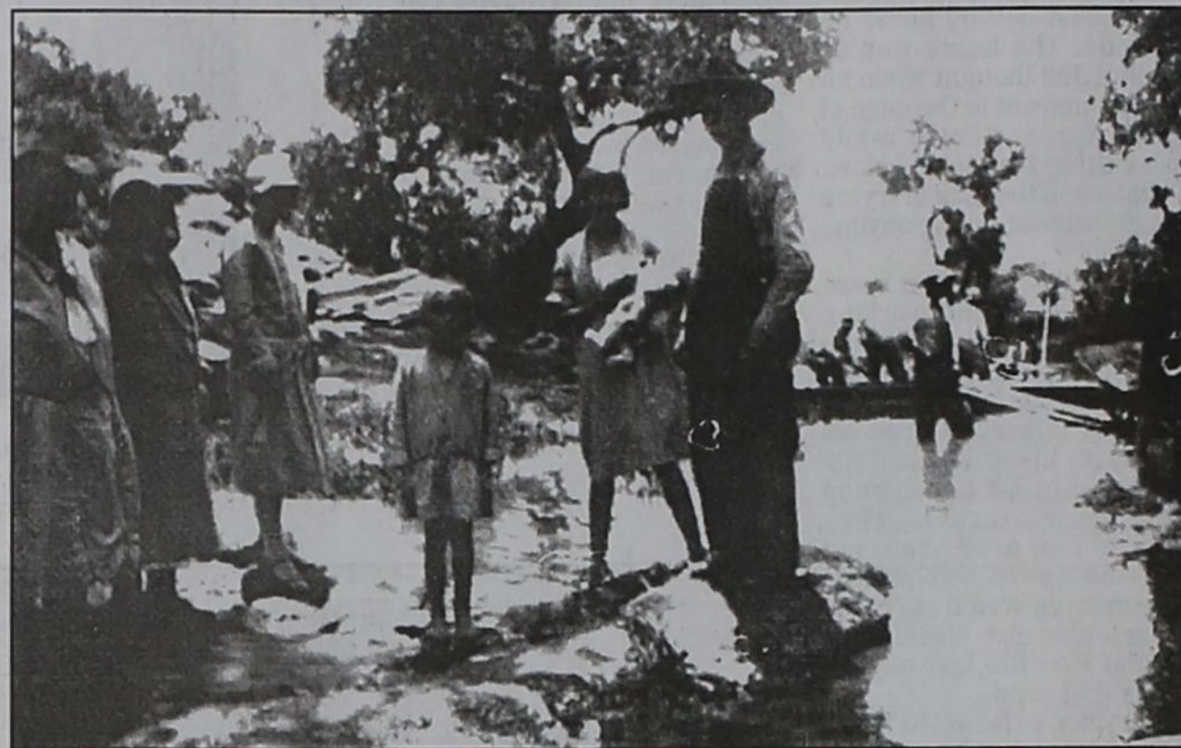
ROARING SPRINGS, MARCH 1929. Rocks were being cleared for the pool to be built.
