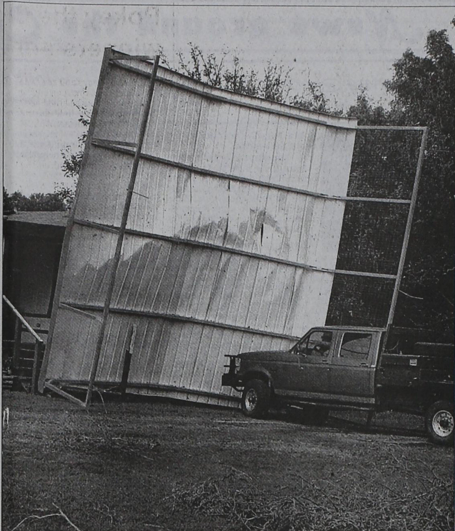
STORM DAMAGE — This carport, belonging to Mr. and Mrs. Don Stuckey in Roaring Springs, was blown over and badly damaged during a storm Sunday night.
