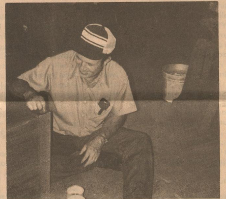
Refinishing Methodist Pew Benches after the church roof fell in.
