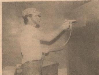
The "landlord," Clay Jameson sprucing up the Tribune's new home.
