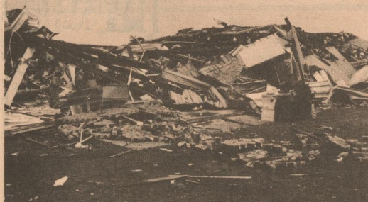
This pile of rubble was all that was left of Motley County School at daybreak, May 2nd, 1984. (Photo by Mary Renfro)
