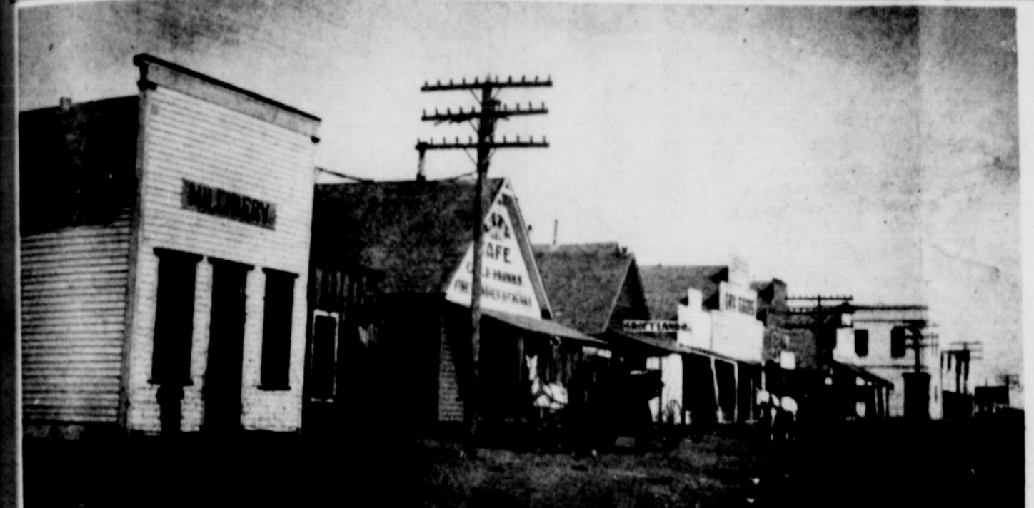
NO STOP LIGHTS were needed on Matador's Main Street more than half a century ago when this picture was made. To aid reader's in orienting the scene, remove the City Cafe and place the Matador Hotel on the exact location, then look north. This was Main Street in 1910, all structures have been replaced including the First State Bank Building, then the only masonry building. At the far right is probably the telephone office, present location of the Tribune building. The two vehicles shown in the picture did not have air conditioning, or two-way radio. Businessmen did not have to pay electric bills, water bills, or sewage bills. Water was carried from windmills (in some instances piped), there were no electric lights, the plumbing was outside. No television, no radio, no sidewalks, no anything much but a place to build the modern, progressive community of Matador.
