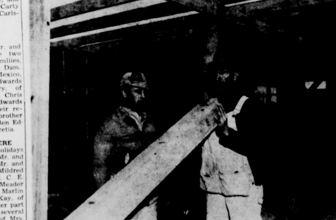
Jack Green, left, has been in the contracting and building business with his father, J. C. (Jimmy) Green, right, since 1938, except for the two years the U. S. Army needed the son as a supply engineer in both the European and Pacific theatres of combat. Released from service he resumed his business association with his father. The firm of J. C. Green and Son is a family affair, with sons Luther, Phil and Richard aiding in constructing buildings from foundation to roof. Richard Green was rated as an expert painter in the army. Phil Green has recently severed relations with his father and brother to accept a position in the First State Bank. Jack Green was born in Matador and attended Matador high school. His father has been a resident of the county since 1910 and entered the building business in 1926. Jack Green was married to Decima Hammersly in 1936. They have four children, Elwanda, Christene, Jimmy and Tommy. This concludes the series of father-son partnerships in Matador unless others are brought to the attention of the publisher. (Photo by Douglas Meador)
