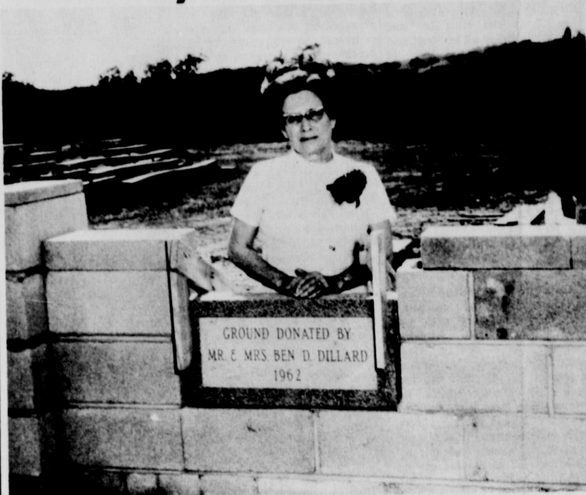
GATEWAY TO HOLY GROUND. Mrs. Ben Dillard stands at the partially erected gate at the entrance of the 43 acres that is the Assembly of God Youth Camp. The camp is about a quarter of a mile from this gate. Volunteer work in building the gate is being done by Rev. Haskell Rogers of Lubbock, who is District Superintendent.
