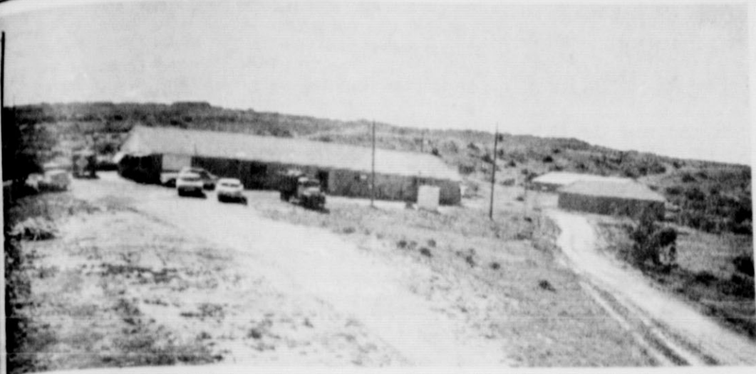
DREAM BECOMES REALITY — Three years ago Mr. and Mrs. Ben Dillard of Roaring Springs deeded 41 acres of land 10 miles east of Roaring Springs to build a youth camp for the Assemblies of God Churches on scenic Tongue River. Today the dream has become a reality, with four masonry buildings, water system and swimming pool. Above photo shows the dining hall and assembly building, with girls and boys dormitories to the right. Picture was made from the water tower looking west. Approximately 1,000 young people from 135 churches will attend this summer. Tribune photo and engraving
