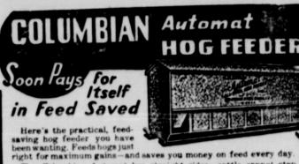
The Columbian Automat has straight sides—cattle cannot step on it and ruin it. Counter-balanced doors open inward as the hog eats; close tightly as soon as the hog withdraws his snout. No chance for chickens to crowd in. Each feed hopper is adjustable to regulate the flow of feed. Bottom of feed trough is slanted so hogs will eat it clean; no crevice or corners where stale or spoiled d can accumulate
