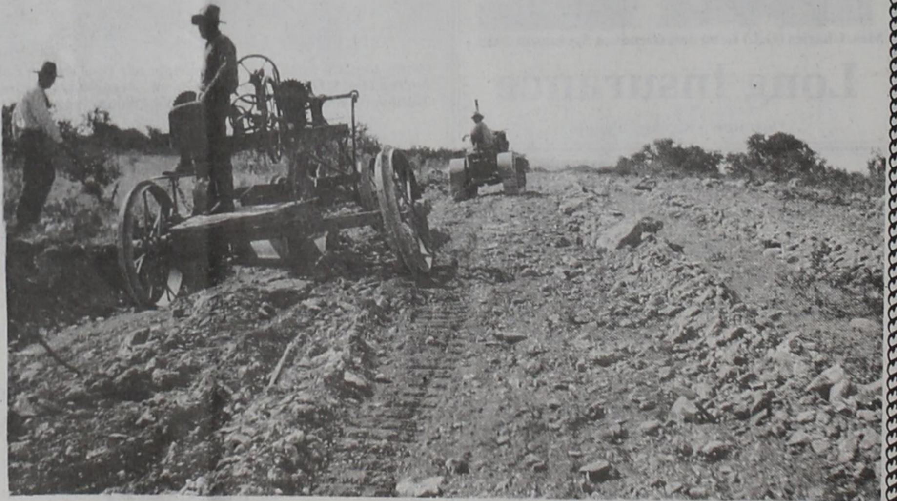
Men at work building roads south of Roaring Springs, 1933-34.
