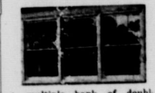
A multiple bank of double hung windows, often used at the end of the living room.
