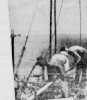
PREPARING TO DRILL a seismicographic shot hole into the floor of the ocean during the search for likely oil-bearing formations which The Atlantic Refining Company is conducting in the tidal waters of Texas and Louisiana. Portable drilling rigs and seismic recording devices are being used.
