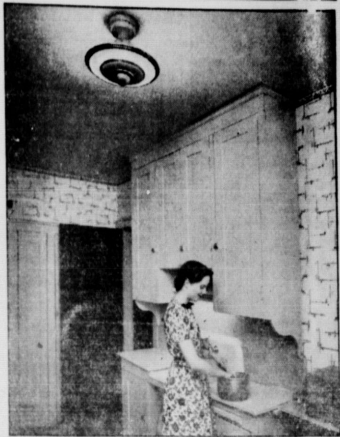
In this re-lighted kitchen, a new "adaptor" unit provides generous cheerful illumination, while above the kitchen sink, a tubular luminescent bulb supplies extra light where it is most needed.
