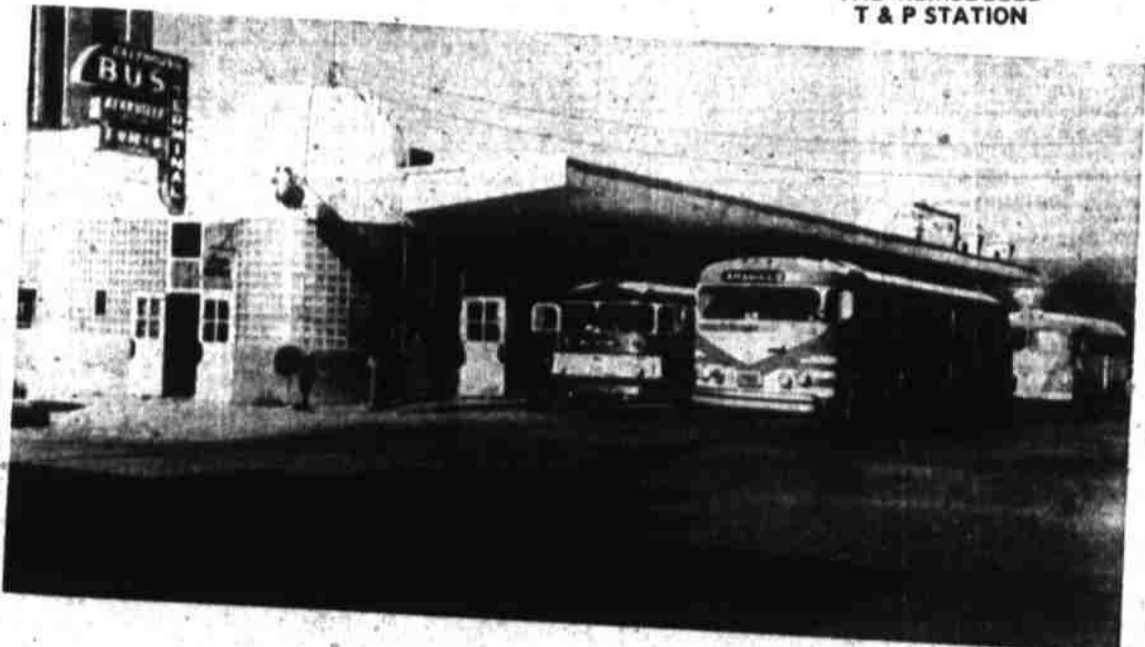
UNION BUS TERMINAL
