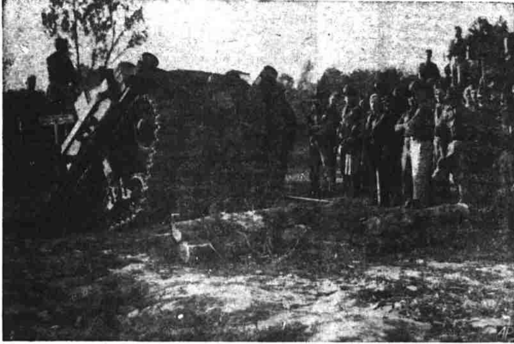
OUT OF THE DEPTHS... OF A TANK TRAP —You can't keep a good tank down—in a tank trap—as can be seen in this view of a tank coming up to level ground during a demonstration at Fort Belvoir, Va. However, there was an embarrassing moment later when the tank, one from Fort Meade, Md., did a flip-flop and landed upside down, after jumping a trench.
