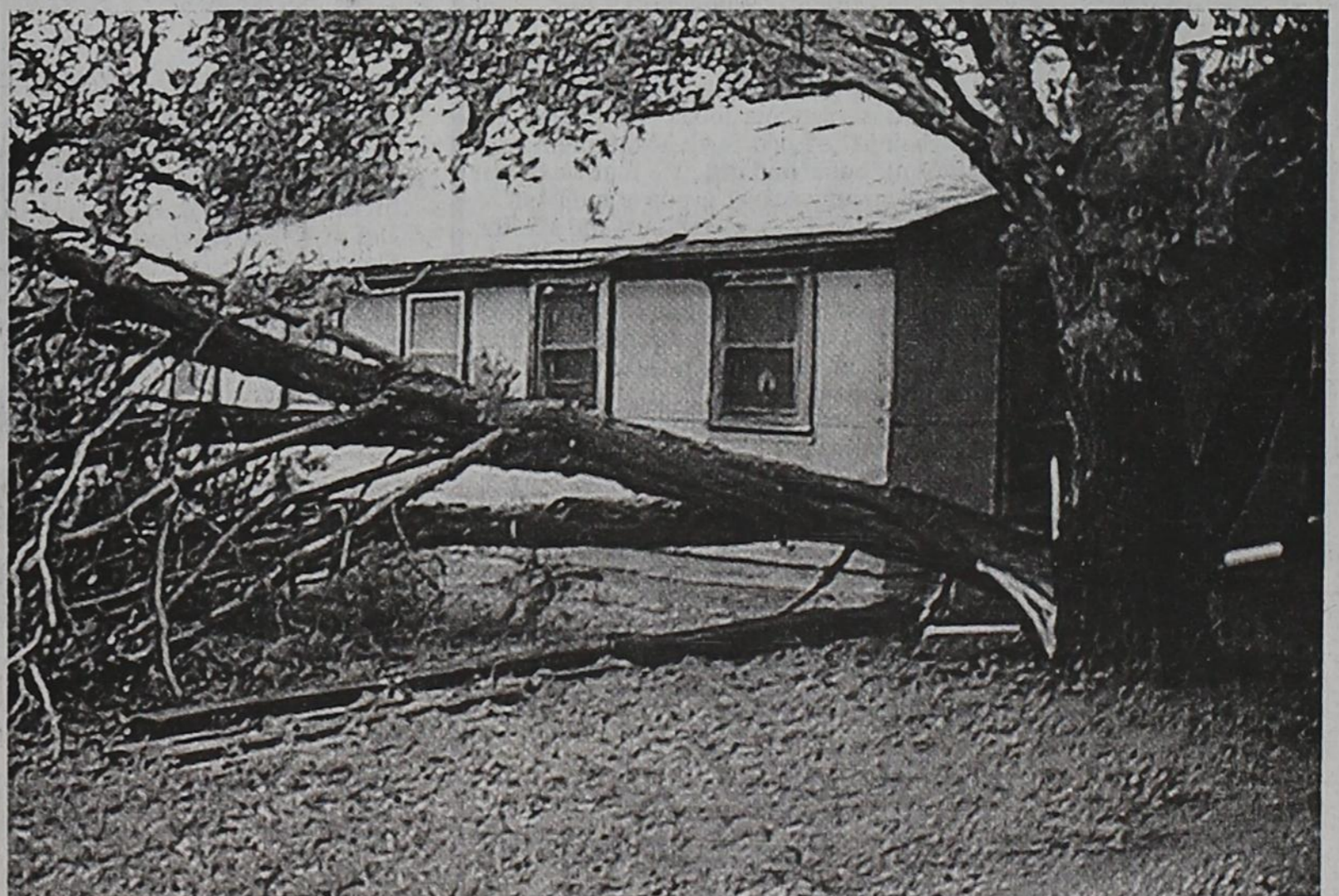
STORM DAMAGE — This downed tree near the home of Paul Gonzalez is only part of the damage residents in north Matador reported from high winds and hail on Tuesday afternoon. Baseball size hail and winds as high as 70 miles per hour were reported. Several homes suffered broken windows and roof damage. Two residents reported broken windshields to their vehicles. Rainfall totals were not available at newstime. See picture on page 4.
