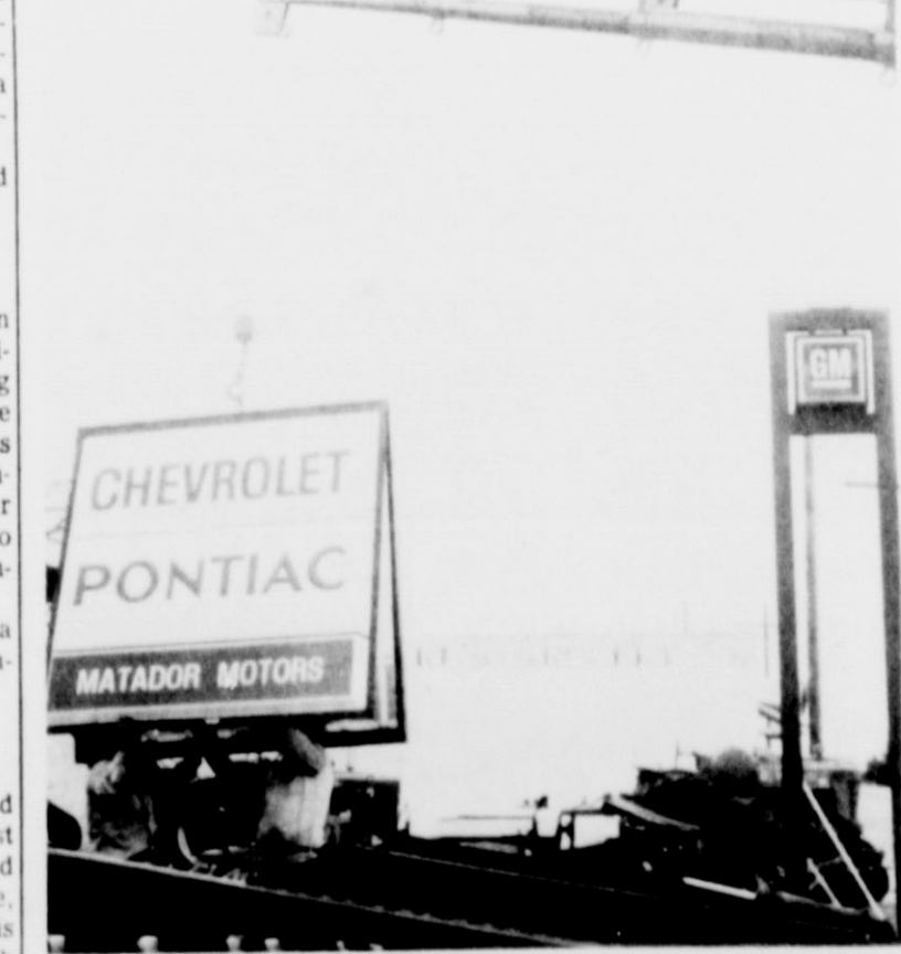
NEW SIGN ON THE ROAD—New Chevrolet and Pontiac sign installed last week for Matador Motor and Implement Co. on Highway 70 (Bailey Street). Photo shows hoist holding sign as workmen make adjustment. The sign is now located on top of the metal (GM) frame at the right. The sign is lighted and visible from east and west. —Tribune Photo
