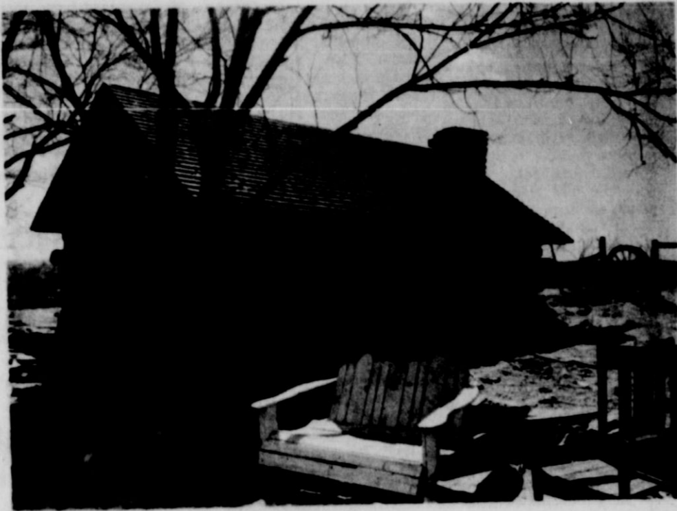
OLD HALF-DUGOUT - built of cottonwood logs at Red Lake Camp in Dickens County in 1890, which is now located at the Ranch Headquarters outdoor museum at Texas Tech University, presented by the family of the late Ennis Moss. It was used as sleeping quarters when extra cowboys stayed at the line camp and was known as "The Dive." (Tribune Photo)
