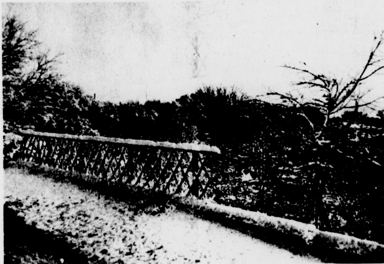
OLD BALLARD CREEK BRIDGE. North Main Steet, Matador
