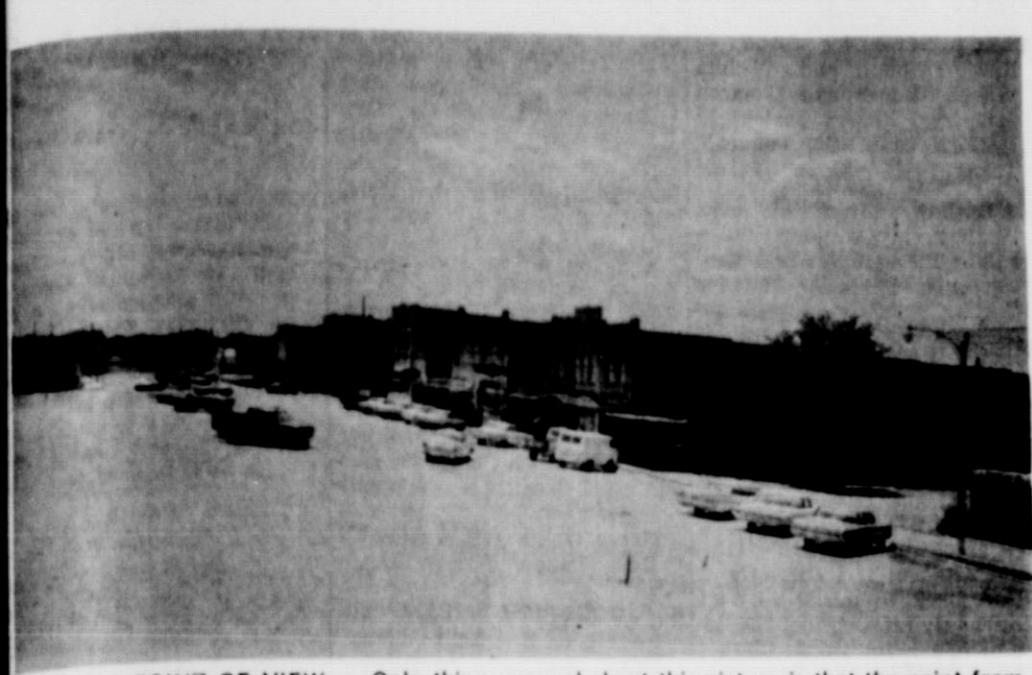
VANISHED POINT OF VIEW — Only thing unusual about this picture is that the point from which it was made does not continue to exist. The photo was made about six weeks ago from the top of old Mission Service Station, which has been demolished and the lot cleared, at the corner of Stewart and Main. View is looking south from the corner on Main Street, with Bob Stanley Pharmacy at extreme left and part of Tribune Building showing at extreme right.
