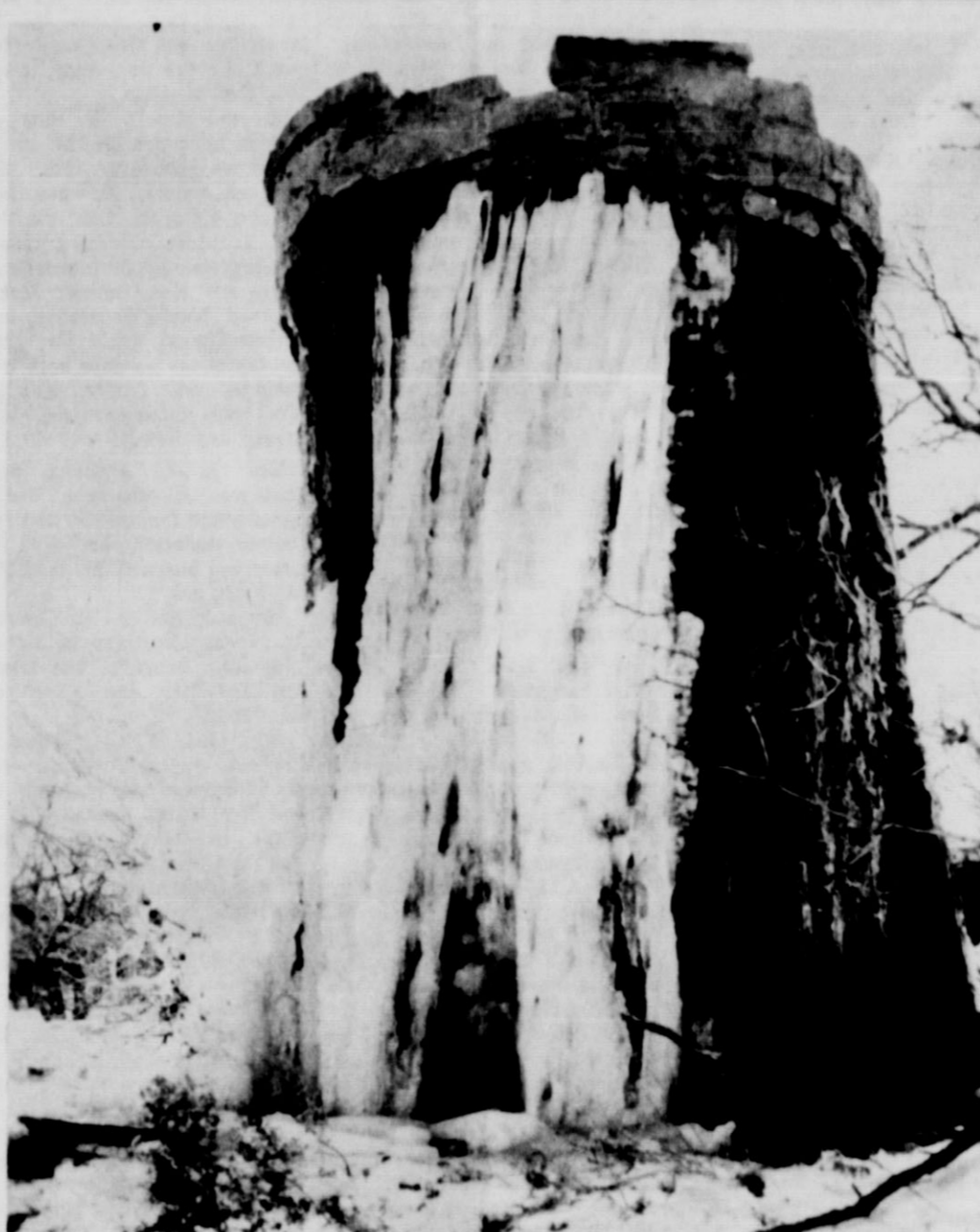
ICE FOR A TALL ONE—The above photo was made last week at the Matador Ranch headquarters here. The Scotch influence is evidenced in the architecture of the water supply reservoir, constructed from native stone more than half a century ago. The pure spring water is piped from West Tank several miles away in the Foothills. When the tank was first built the water was obtained at historic Ballard Springs, a few hundred yards away. The big icicle was formed last week when the tank overflowed during sub-freezing weather. Much colder weather has prevailed in the past several days and some of the snow which fell over ten days ago is still on the ground.
