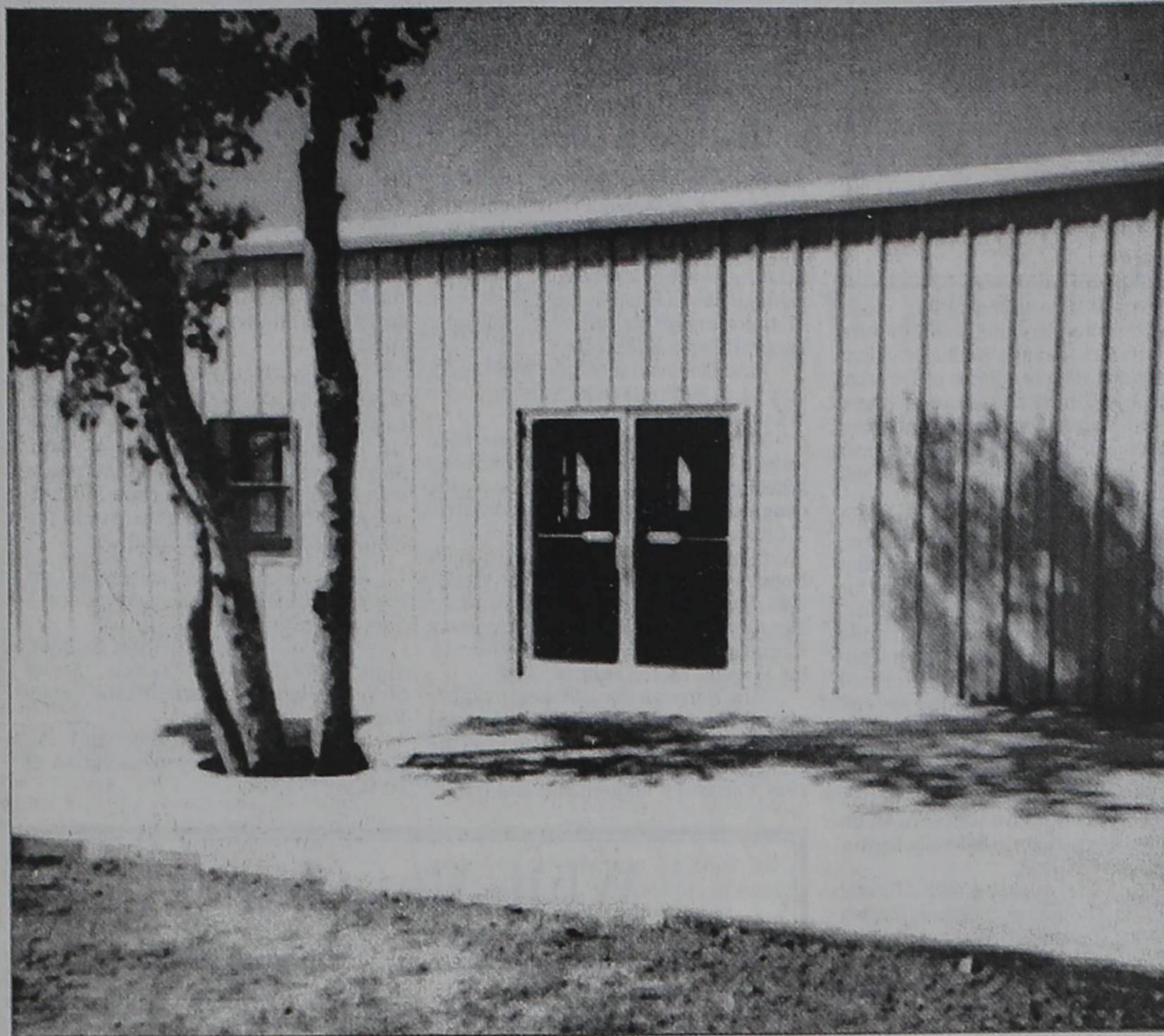
ROARING SPRINGS COMMUNITY CENTER — The newly completed Roaring Springs Community Center is now ready for use. This week it is being put to good use by the Community Volunteers sponsored Kids' Camp. The center is a project of the Roaring Springs Volunteers and will be available for use by various clubs and organizations. The center will also be available for family reunions, classes or seminars. For information contact any Community Volunteer member.
