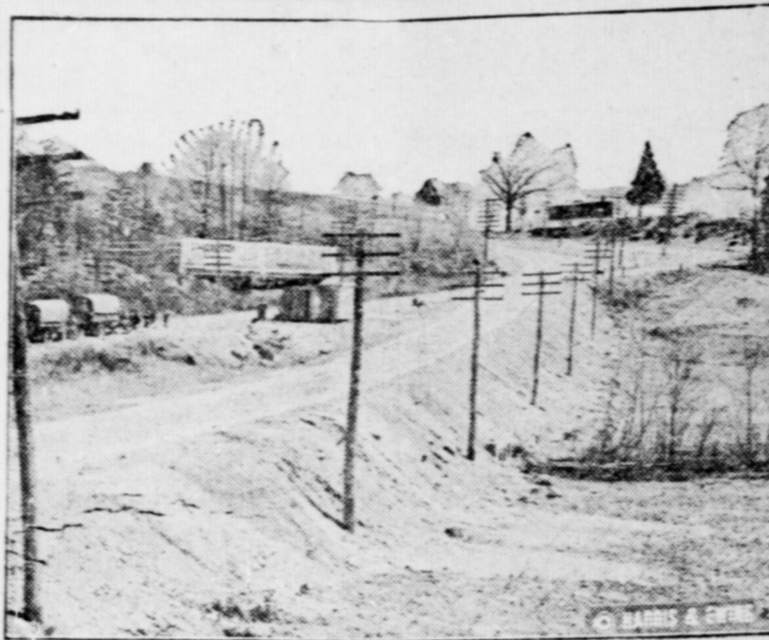
Baltimore and Washington motorists who have had occasion to drive between those two cities, are greatly pleased that "Dead Man's Curve" has been removed. The cutoff in the right-hand corner of the photograph was the danger spot. Many cars running at high speed, unable to take the curve, plunged into the field at the right, in many cases resulting in death and injury.
