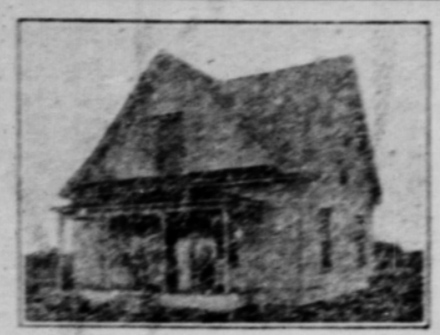
FINISHING A PLAINS HOME
