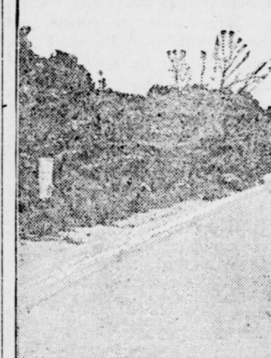
Experiment Road of Vitrified Brick for Paving Country Roads at Chevy Chase, Md.—Finished Pavement in Service.
