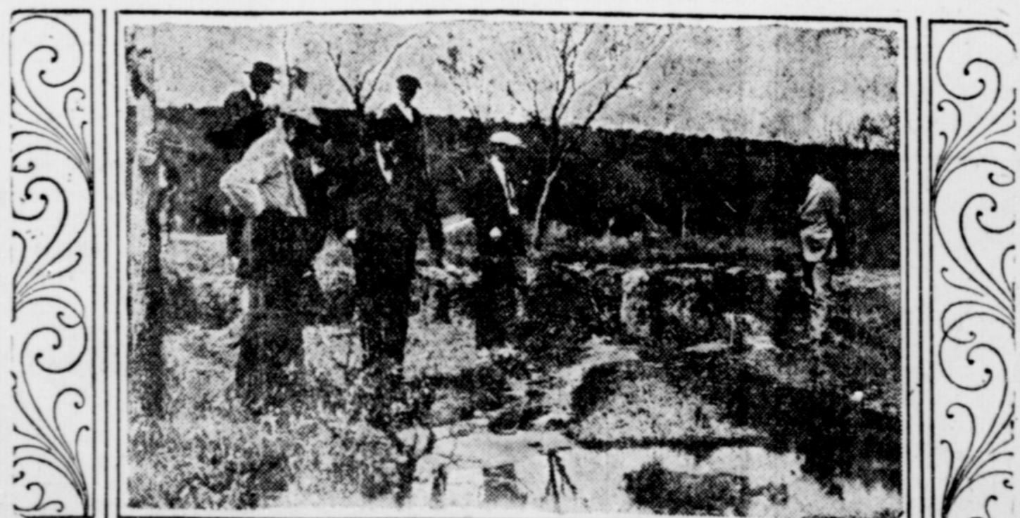
Nearby creek was dammed to take care of the precious fluid until pipe line connections could be made.
