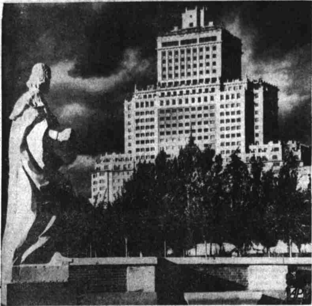
OLD LOOKS UP TO NEW — Statue of ancient Spanish King in palace gardens contrasts with 25-story apartment-hotel skyscraper nearing completion in capital city of Madrid.
