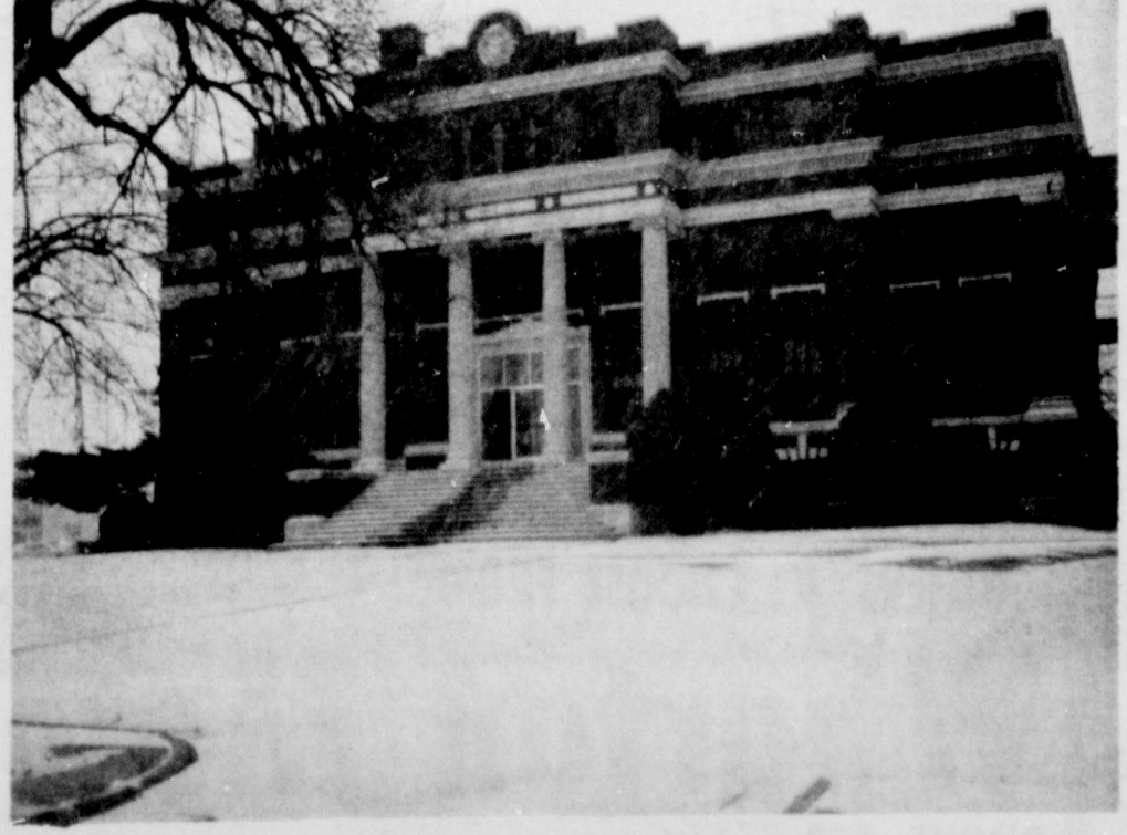
TAHOKA DOES RECEIVE SNOWFALL AS EVIDENCED IN THIS PICTURE OF THE LYNN COUNTY COURTHOUSE, AS SNOW BEGAN FALLING TUESDAY AFTERNOON.
