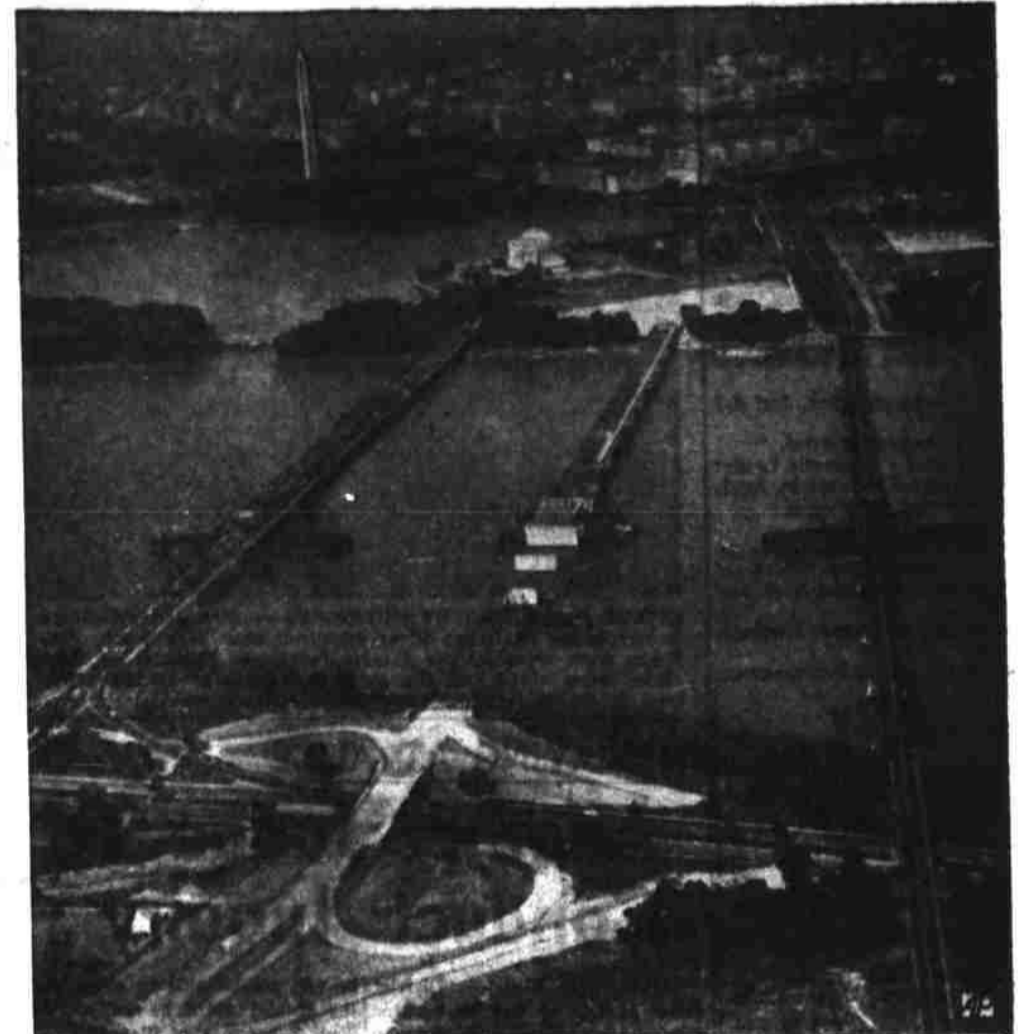
WASHINGTON BRIDGES —The new Washington 14th Street bridge is seen from the Virginia side between older bridges. Cloverleaf at bottom will channel traffic to Mt. Vernon Highway.
