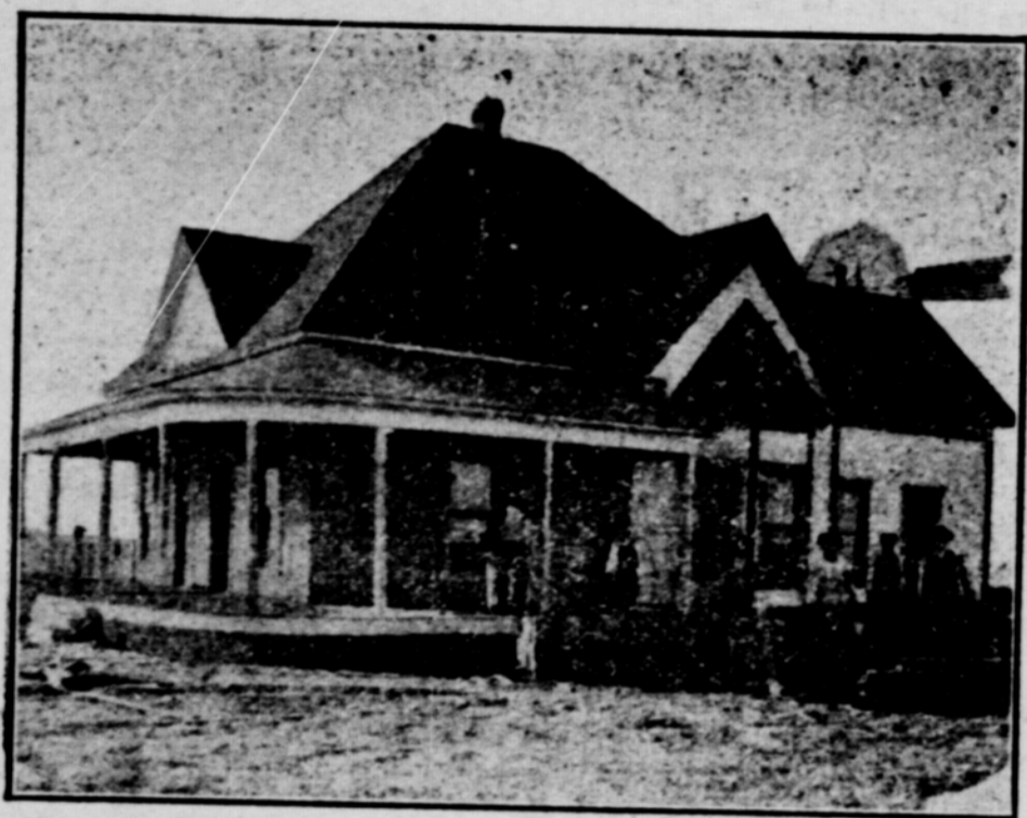
A. L. LOCKWOOD'S HOME, NEAR TAHOKA.
