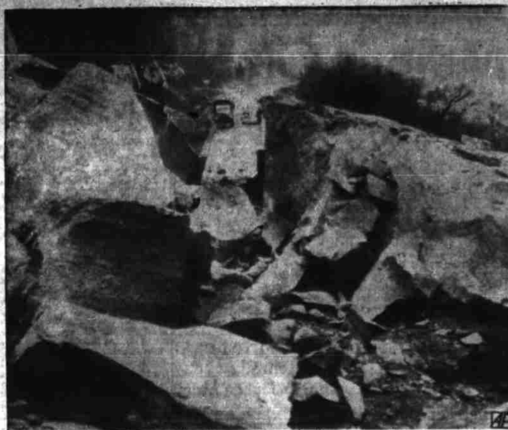
ROAD CLOSED—Tons of rock covered 200 feet of state highway 7, Skyline Drive, near Marietta, Ohio. The rock slipped over the road, which was cut through almost solid rock a few years ago. No one was injured. Highway engineers said the road would be closed for two or three days. (AP Wirephoto).
