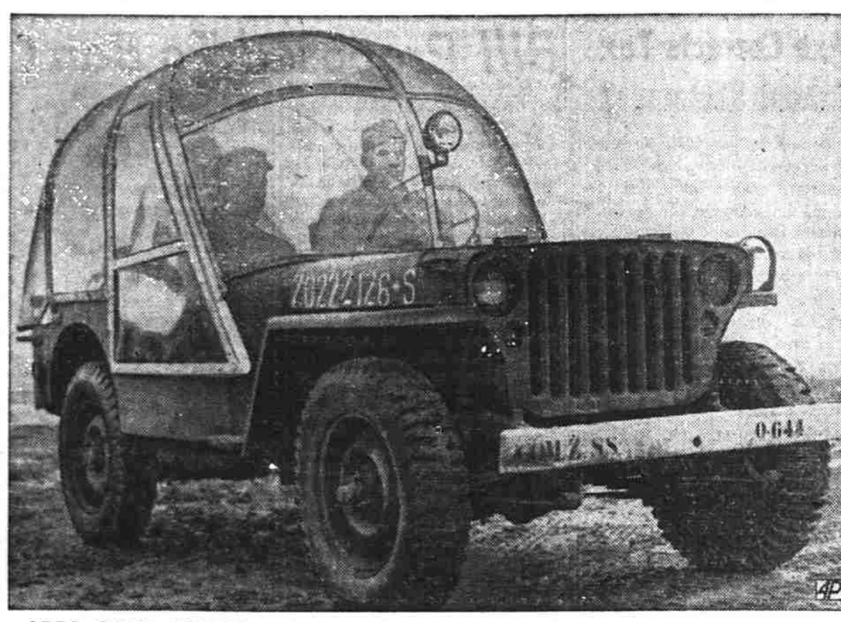
JEEP GETS COVER — Yanks at an ordnance depot in the ETO ride in a jeep which they covered with a plastic tear-drop enclosure made from salvaged material.
