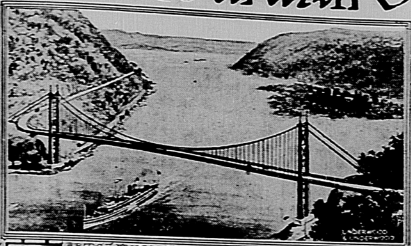
BRIDGE FROM WEST BANK OF HUDSON
