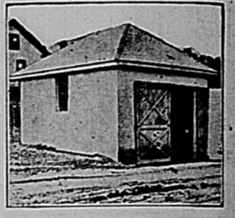
Garage Built of Concrete Blocks.
