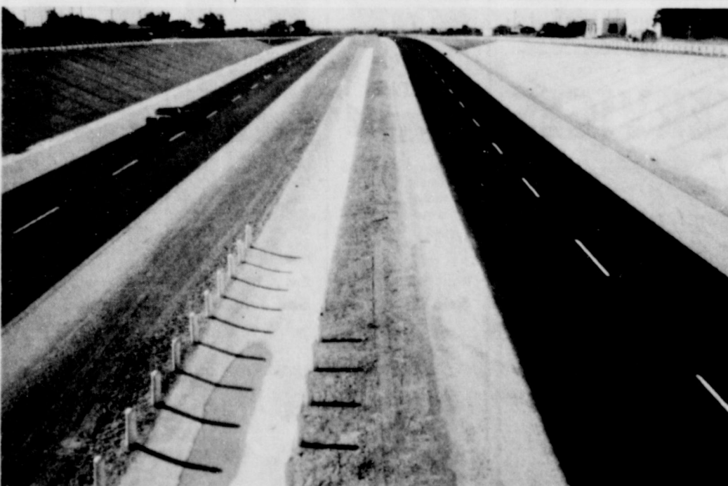
FAST AND NEW are the words to describe the new Highway 87 Tahoka bypass, officially opened last week. The opening has reduced through traffic downtown and also, a trade drop at the local service stations. NEWS Photo
