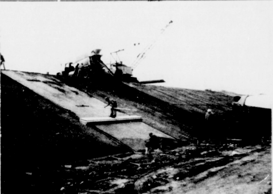
TONS ON CRETE AND BACK-BREAKING WORK GO INTO THE JOB OF POURING AND FLOATING THE RETAINING SLABS ON THE NEW HIGHWAY FILLS. STAFF PHOTO
