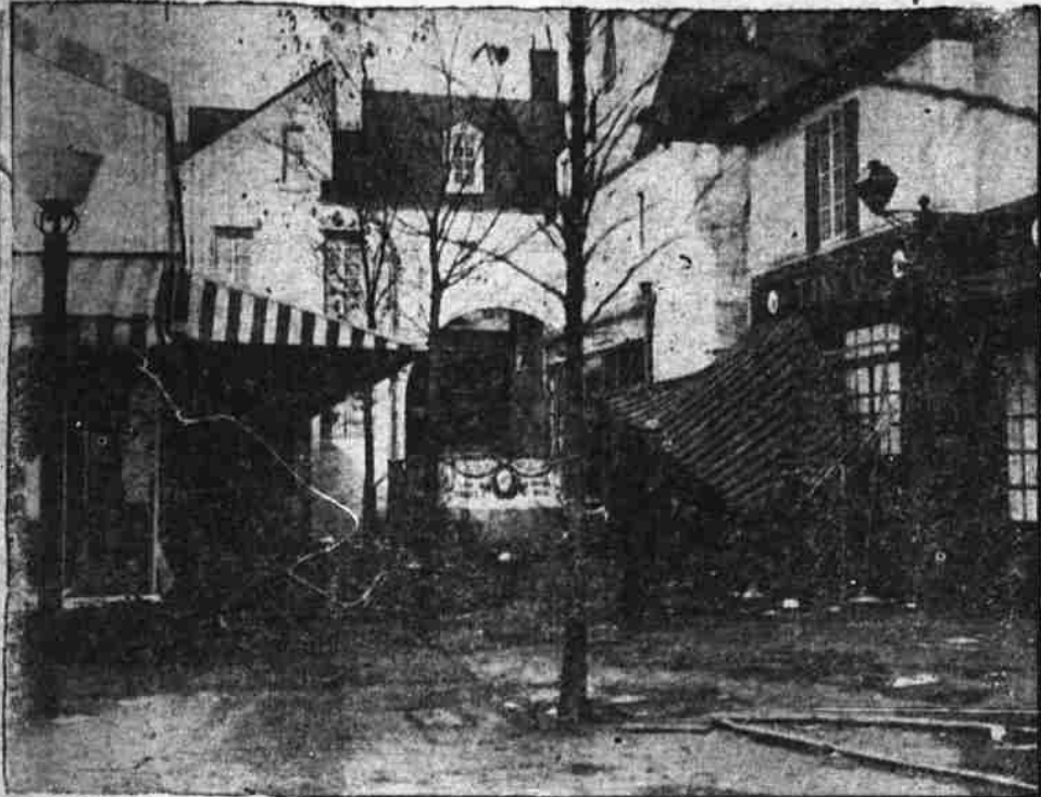
Debris littered the "Streets of Paris" at A Century of Progress in Chicago after "last night's" had run riot, wrecking $150,000 worth of concessions and exhibits and tossing policemen into the lagoon. More than 300,000 persons jammed the grounds on the last day of the two-year exposition. (Associated Press Photo)
