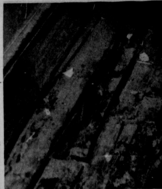
ROTTING FLOOR -- This floor in the junior high gym is part of the repair work needed in the Junior High School building.
