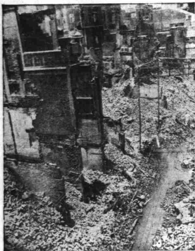
AFTER INDIA RIOTS — Blasted and burned buildings line street in walled city of Lahore, India, after riots between Moslems, Hindus and Sikhs over the Indian partition plan. Punjab Assembly in Lahore later approved plan.
