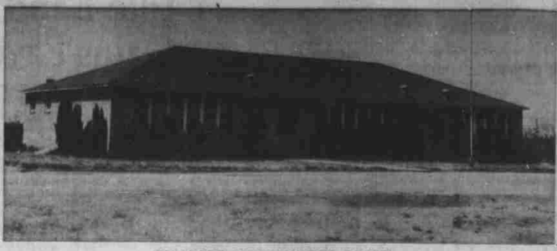
COLORADO CITY'S BUFORD SCHOOL. Idle building an issue in bond election
