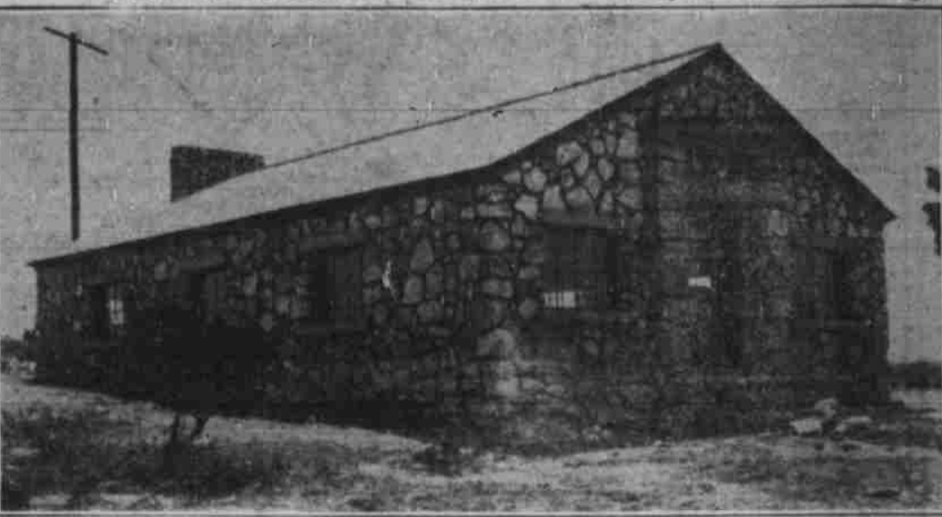
Made of native stones gathered a few yards from where it stands in the city park, this building was provided as permanent Boy Scout headquarters five years ago. It is the center of the annual Jamboree of the Buffalo Trail council.
