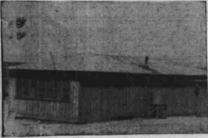
The only frame structure in the entire Big Spring school system is the two-room negro ward school. Although the building is a recent acquisition, a negro school was provided for the city the first year the system was incorporated.
