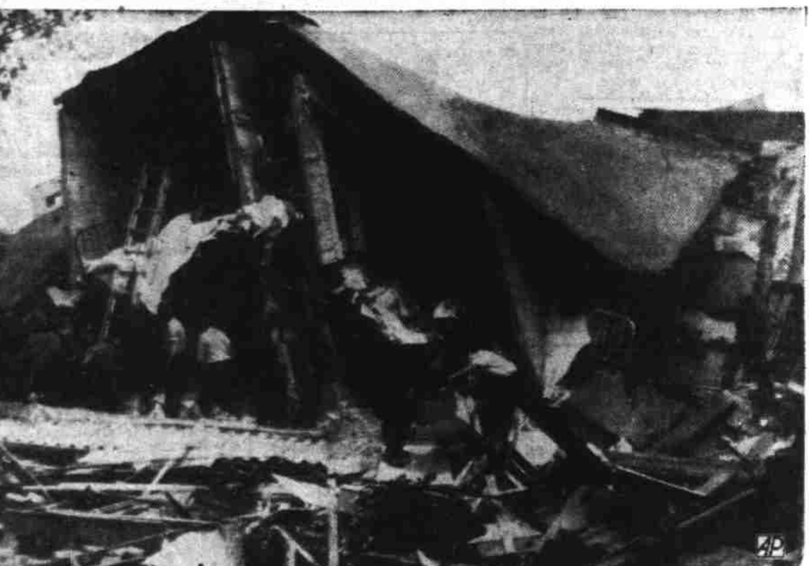
EXPLOSION WRECKS APARTMENT BUILDING—Walls were blown out and rooms exposed, as shown here, when an explosion wrecked a two-story apartment building in Denver, Colo. Police Capt. L. C. Morlan said two persons were killed and seven or more injured. (AP Wirephoto).
