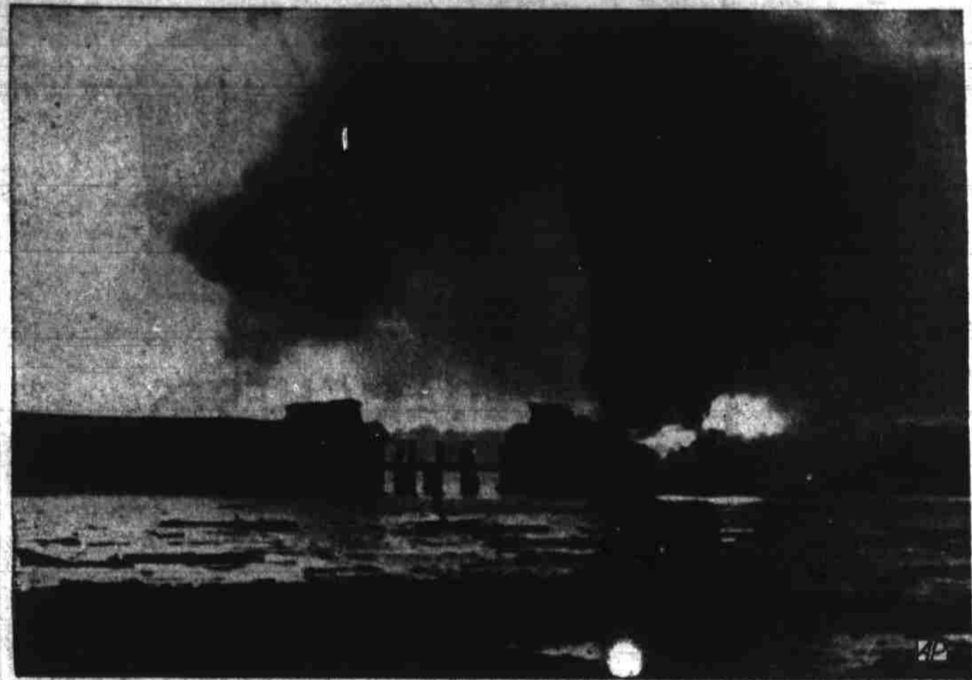
BLAST SCENE—Shown is a general view of the scene where four munition-laden barges exploded at the South Amboy, N. J., docks killing several persons and injuring nearly 300. Fire is shown still blazing on the barges and dock. Officials said damage to homes and stores alone would run to more than $1,000,000 (M). (AP Wirephoto).
