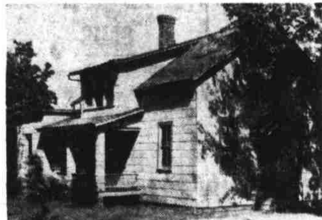
But a dormer window upstairs, a new roof and asbestos siding made it neat.
