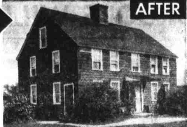
Spruced up with shingle siding and a new roof it revealed its hidden value.
