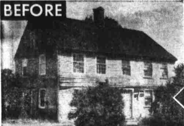
This big house was sadly neglected, but its defects could be easily remedied.
