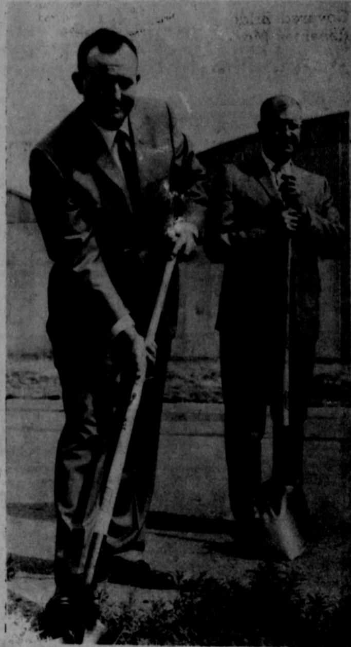
BREAKING GROUND--Tri-State Bakery President R. C. (Pete) Fisher of Spearman turns the first shovel of dirt as construction began last week on the new Tri-State Bakery in Amarillo. In the background is M. W. Sweet, Bakery Manager.
