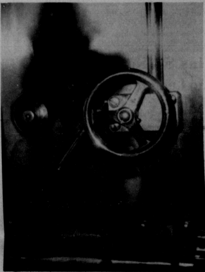
IT HELD— This door to the vault of the Gruver State Bank was damaged by a burglar's cutting torch, but it withstood the attack by cutting torch and sledge hammer.
