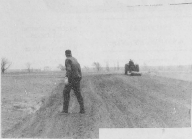
New T-Box at Course!
