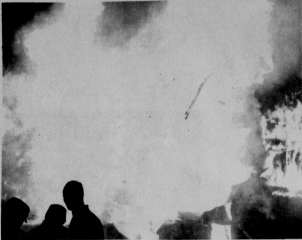
BALL OF FIRE --The first headhouse on the McLain elevator turned into a ball of fire when it collapsed about 11:30 p.m. Sunday. The fire was discovered about 11 p.m. and firemen from Spearman, Gruber and Perryton fought it for two hours before bringing it under control.
