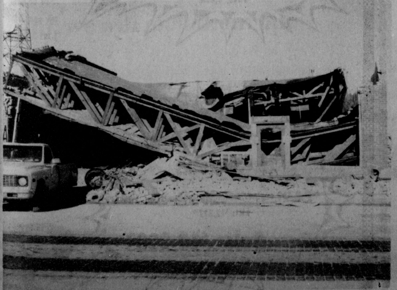
WHITE'S AUTO STORE clean up continues...Perry Washington is in the process of removing
